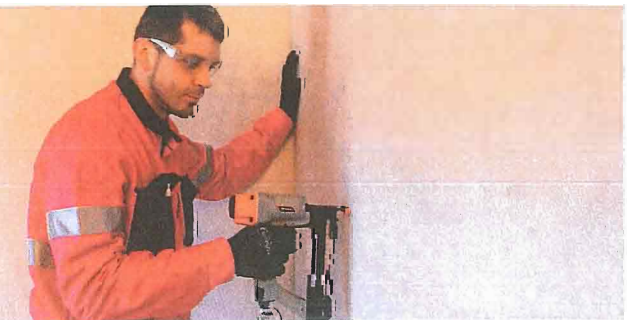
Picture No. 9: Nailing, stapling.
